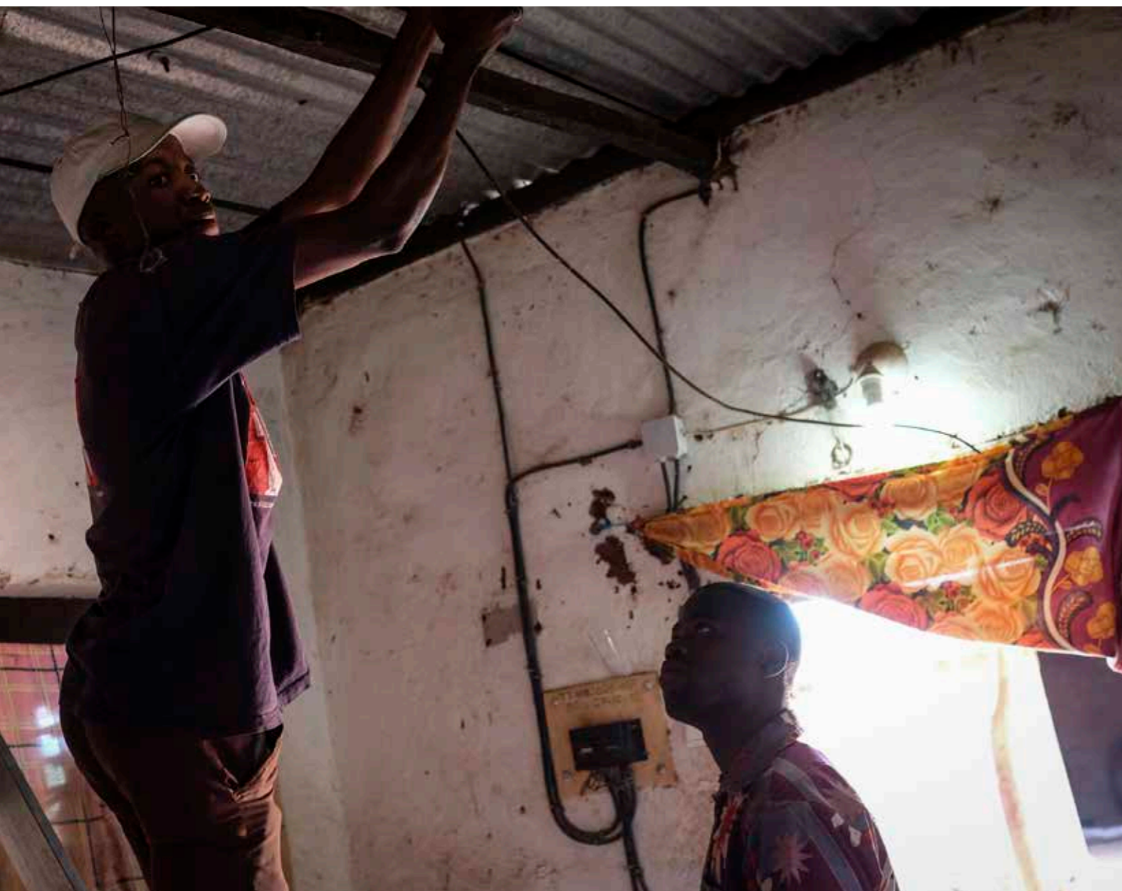
Technician of Yeelen Ba installing light in a household in Kourinion (Burkina Faso)
